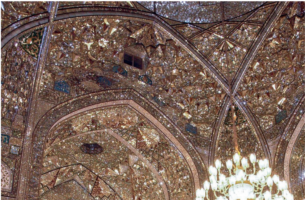
Figure 18. Close view of Dar-al-siadeh terrace-Razavi Haram, 1300. Photo by Masoud Nozari.
